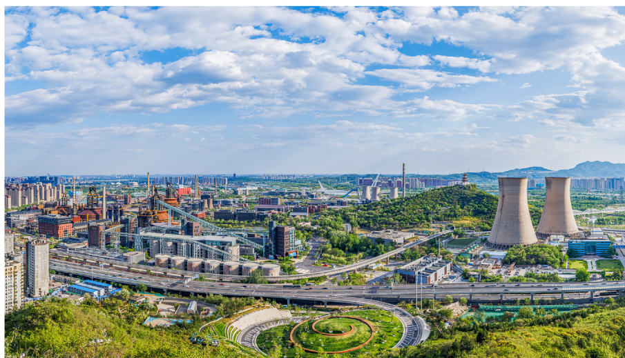
Fig. 2. Shougang Park has a rich history of over 100 years and is considered one of China's earliest and most significant modern steel enterprises. It played a crucial role in the country's industrial and metallurgical development. In 2010, the primary steel production process of Shougang Park was permanently shut down to improve Beijing's clean air after the city won the bid for the Summer Olympics. Despite this, the park was not demolished and remained idle until 2016, when it was repurposed as the first theme cultural park in China to feature steel industry cultural relics. This transformation was based on protection and utilization, and it was made possible by the entry of the Winter Olympics Organizing Committee. Today, visitors can explore and learn about the rich cultural heritage of China's steel industry at Shougang Park. (Photo by Visual China Group).
