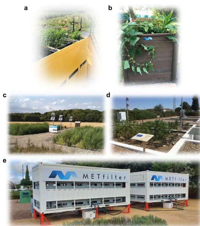
Fig. 5. Different implementations of METland® treating real urban wastewater. a , Modular METland® treating 25 \text{ m}^3 \text{ d}^{-1} at Otos municipality (Spain). b , Modular single-house system treating 1 \text{ m}^3 \text{ d}^{-1} . c , Constructed METland® treating 20 \text{ m}^3 \text{ d}^{-1} at Orby (Denmark). d , Constructed METland® treating 5 \text{ m}^3 \text{ d}^{-1} at Carrion de los Céspedes (Spain). e , Containerized modular METland® operating in series for treating municipal wastewater at Seville (Spain).
